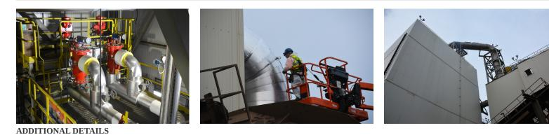
A new emissions control system is being installed at the Schnitzer Steel Industries scrap metal shredding facility in Everett, MA. Methuen Construction is providing the labor, materials, equipment, tools and supplies to install steel framed enclosures, support structures, procured equipment and associated architectuaral, mechanical, and electrical work in support of the shredder emissions control project.
