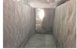
Before beginning any work to repair the tunnels leading to the Enel Hydro turbines, the sections of the collapsed tunnels had to be shored up, which required special safety procedures. This project was in two phases, first to provide tempoary repairs to the collapsed tunnels, and secondly to provide a permanent solution for the tunnels. Methuen Industrial Services provided the skils and experience to address this serious situation.
