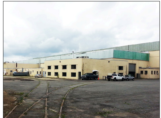
Existing Building - July 2015 - Pre-construction
