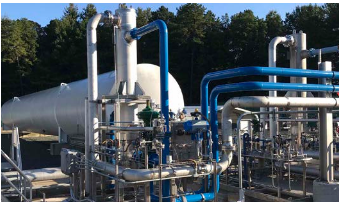
Liquefied Natural Gas Vaporizer Skid, Whately, MA
